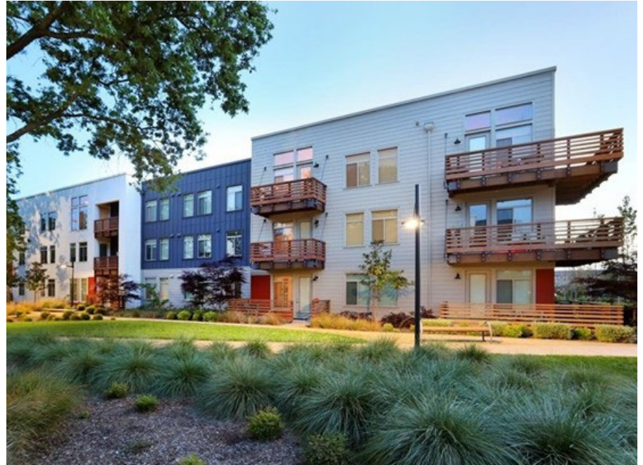
Annadel Apartments, Santa Rosa (24 units/acre)
